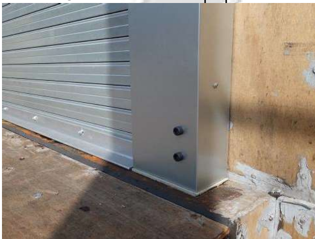
A3. 2 Locking bolt on both roller shutter guides
